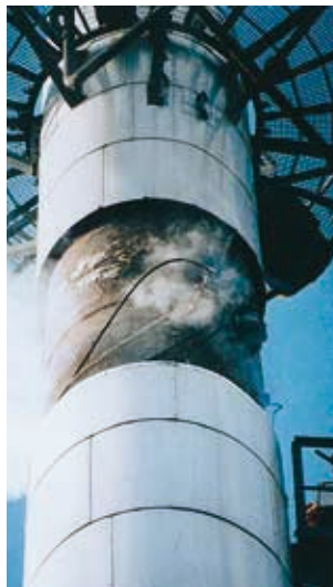
Demolition of double-walled steel structures
