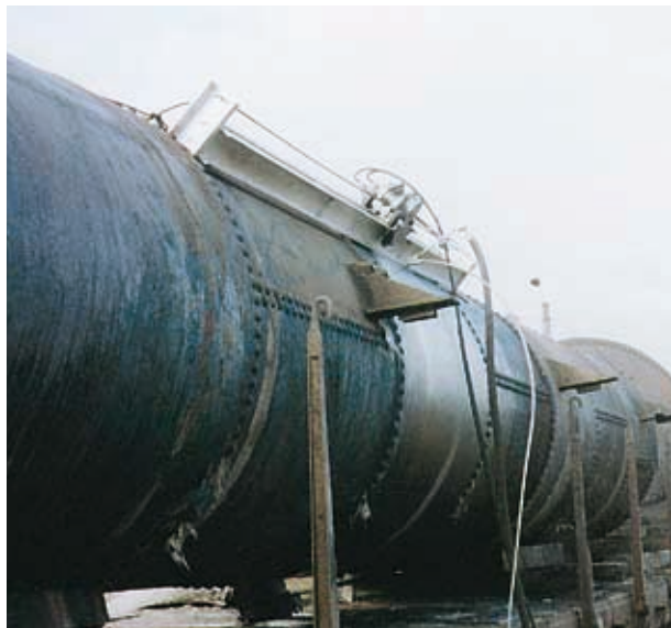
Cutting openings in large storage vessels
