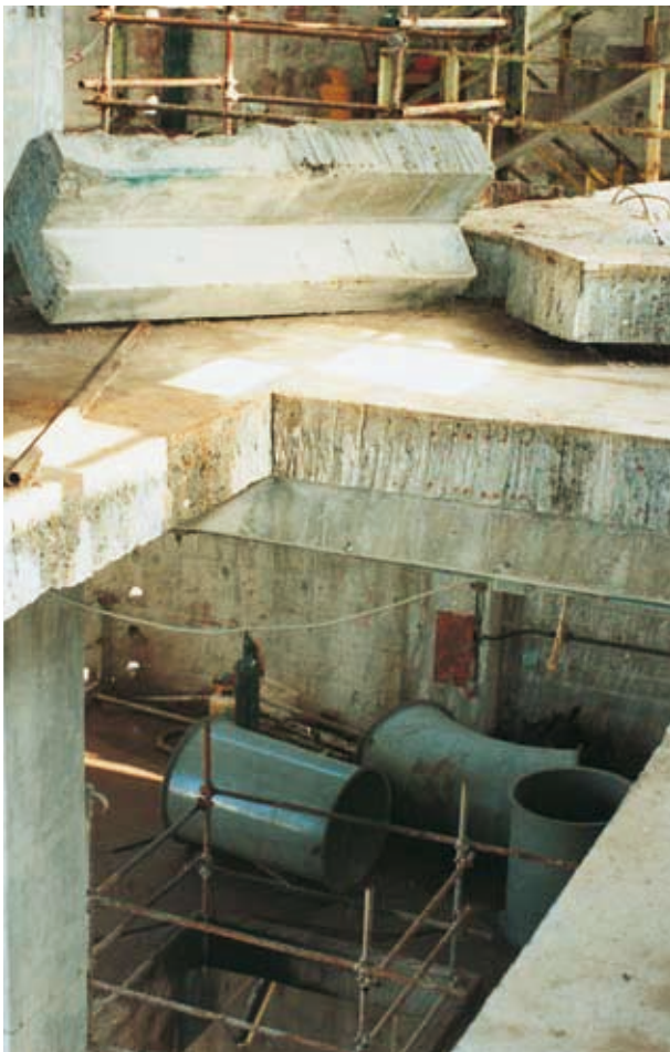
Partial demolition of heavily reinforced concrete ceilings
