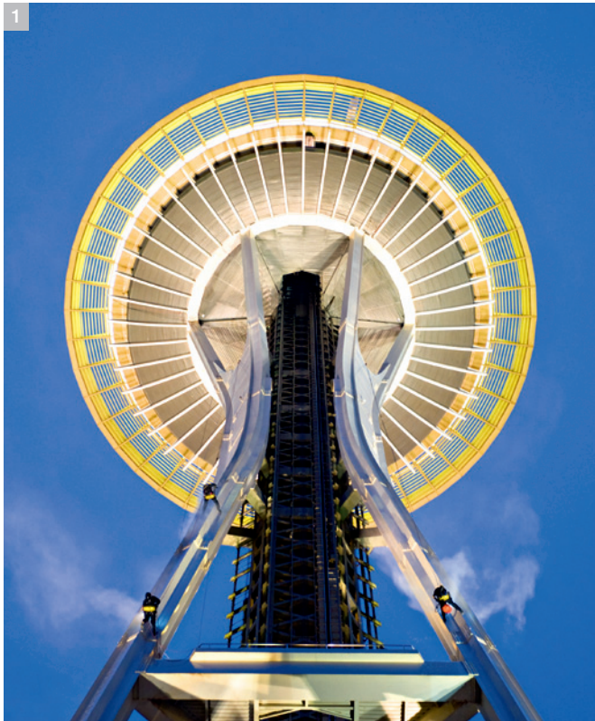
1 Seattle's highest building: The Space Needle A Kärcher team pressure-washed the structure up to a height of 184 m. The job took eight weeks, working only at night.
