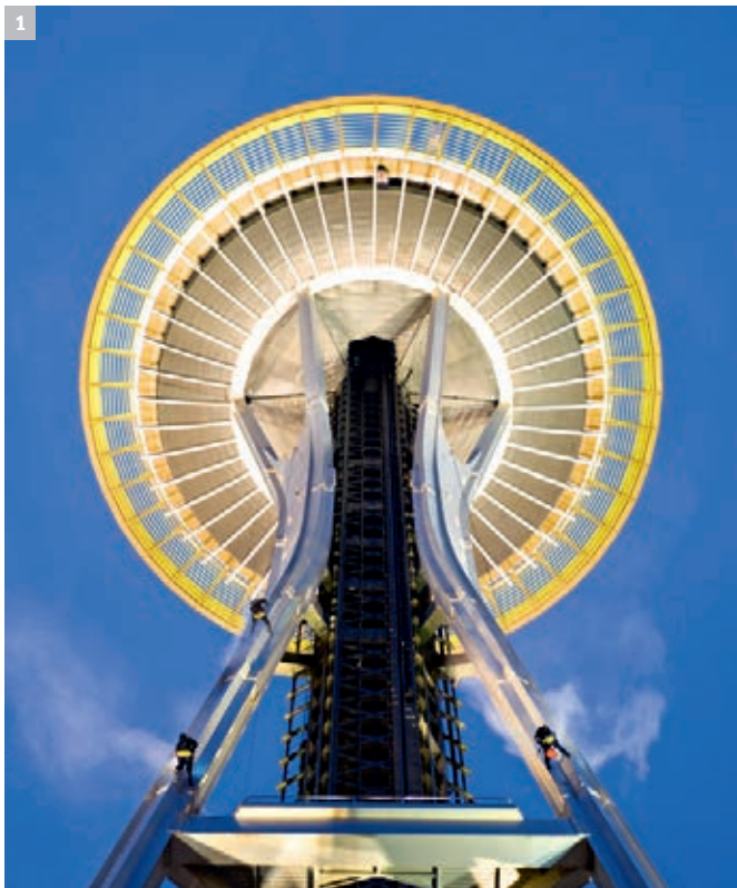
1 Seattle's highest building: the Space Needle A Kärcher team pressure-washed the structure up to a height of 184 m. The job took eight weeks, working only at night.
