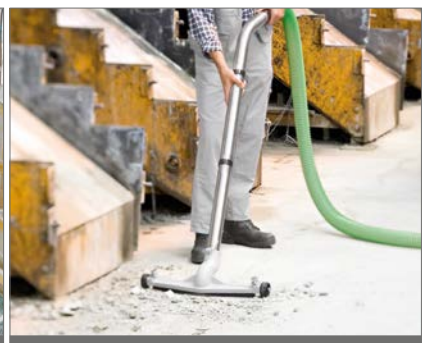
Vacuuming mineral residues, for example concrete
