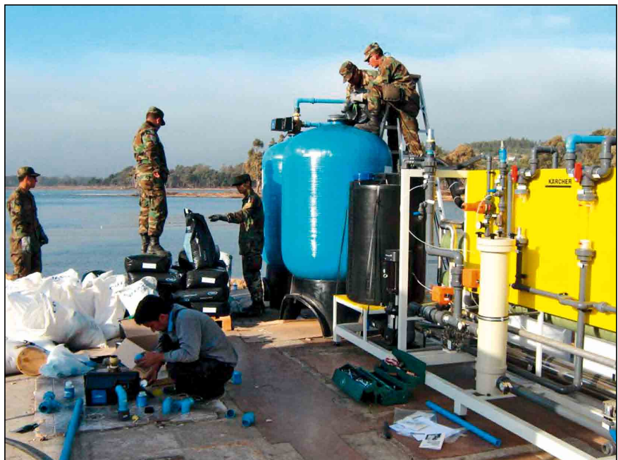
Chilean aid workers set up the Kärcher water treatment plant together with Emasa staff.
