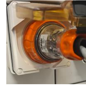
Step 33 Insert the plug of the connecting cable into the socket and turn power on to charge
