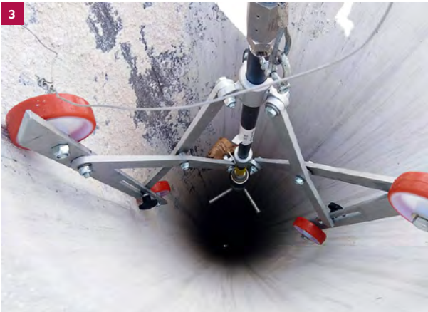
1 2 The EcoMaster D 250M Classic, with an operational pressure of up to 3,000 bar, offers the necessary performance for the removal of concrete and coating. 3 Pipe cleaning
