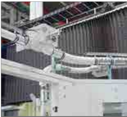
● Pipeline system with electropneumatic shutter and electric control units
