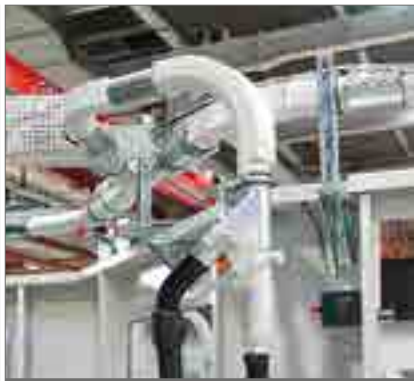
● Pipeline system with electropneumatic shutter and electric control units
