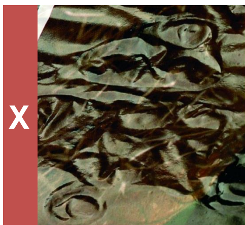
Figure 7: Bubbling due to a sheet that is too damp. [10]
